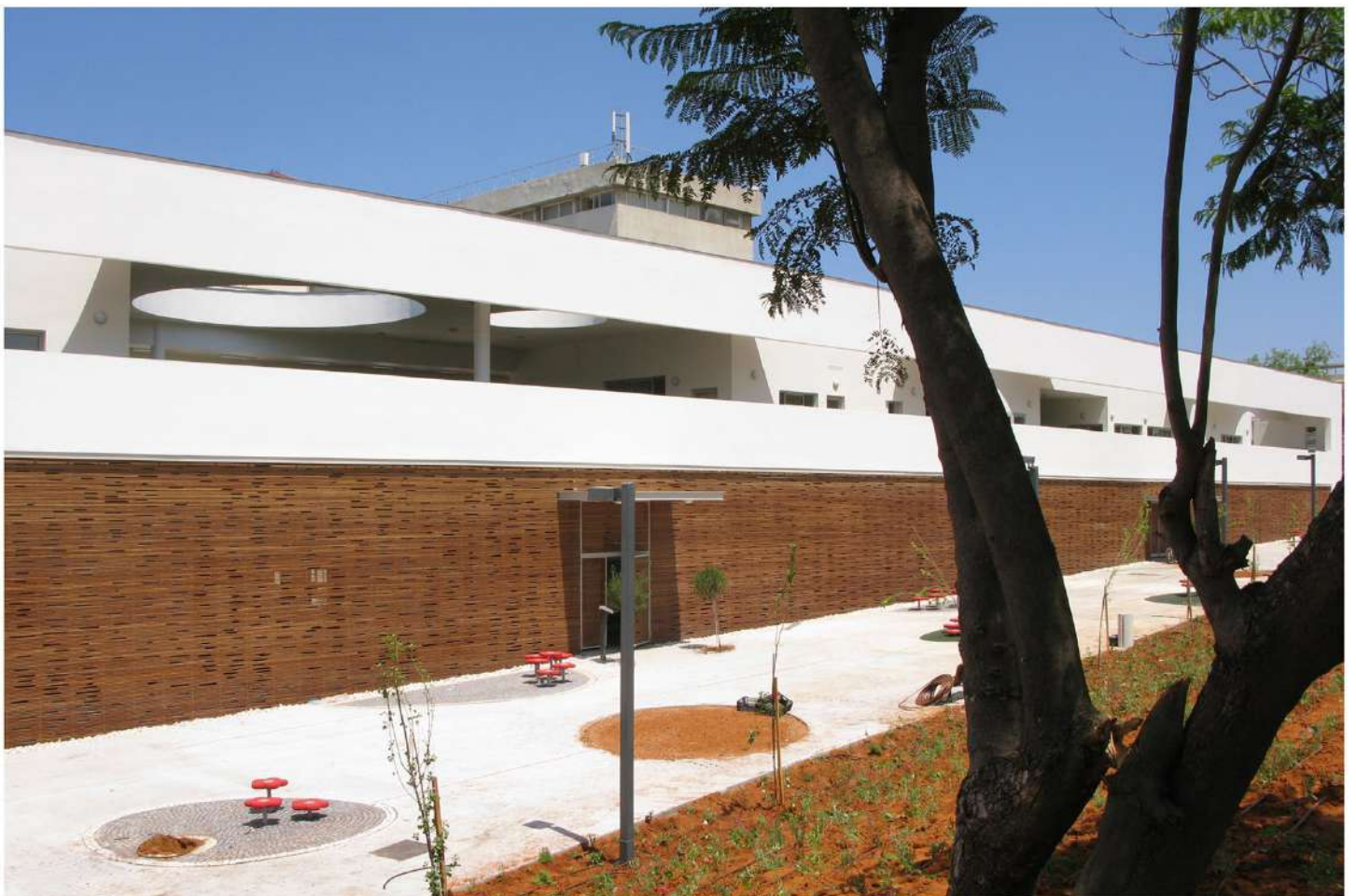
The eastern façade and the kindergartens' entrance: a contemporary variation of the Tel-Avivan brise-soleil tradition
